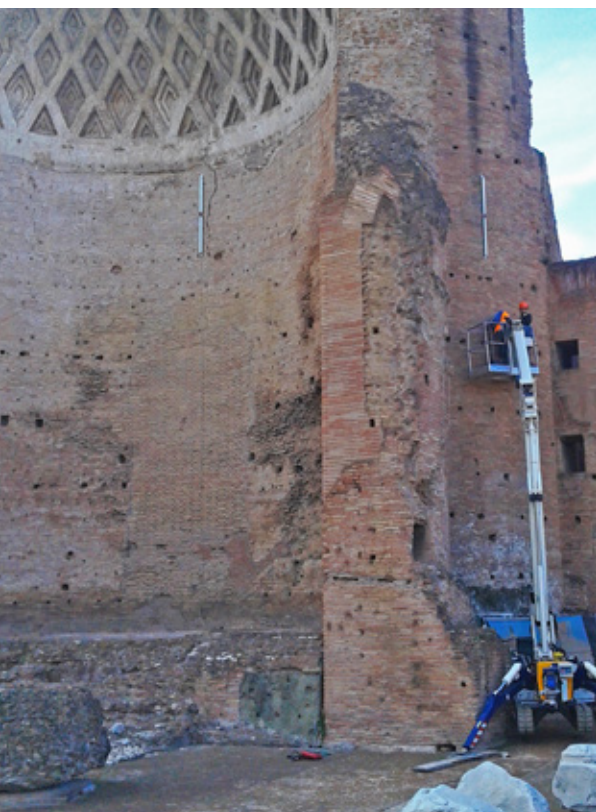
Tilt beam installation on Maxentium Basilica
