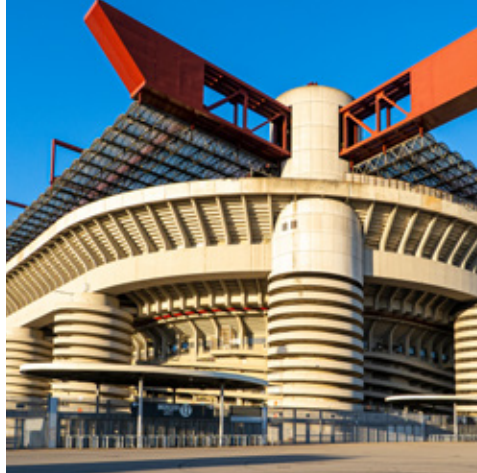
Roof top dynamic monitoring with Tiltmeters, San Siro Stadium, Milan - Italy
