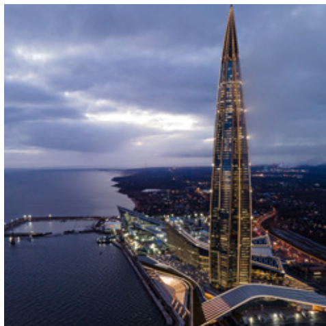
Foundations and building monitoring, Lakhta Tower, Saint Petersburg - Russia
