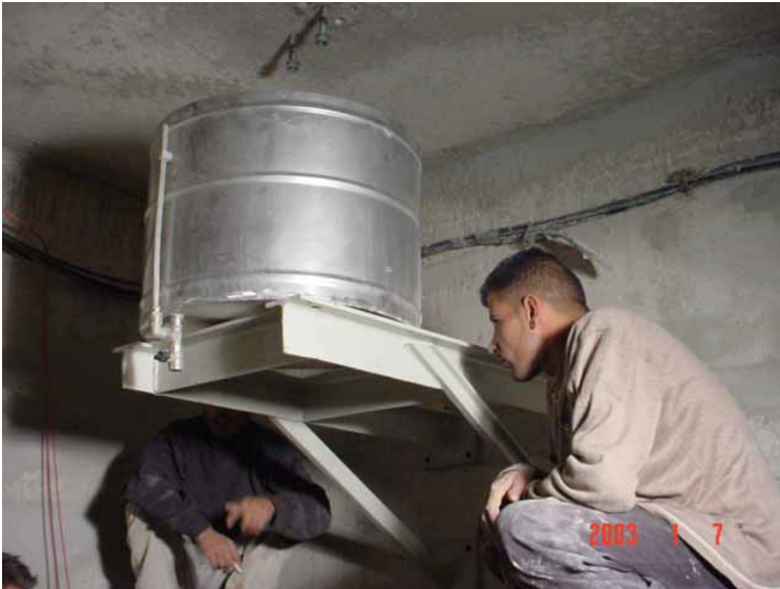
Installation of inverted pendulum tank
