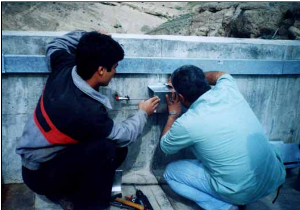
Installation of mechanical jointmeter
